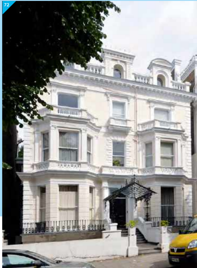
72. 75 Holland Park London UK Communal Boiler Systems Compliance
